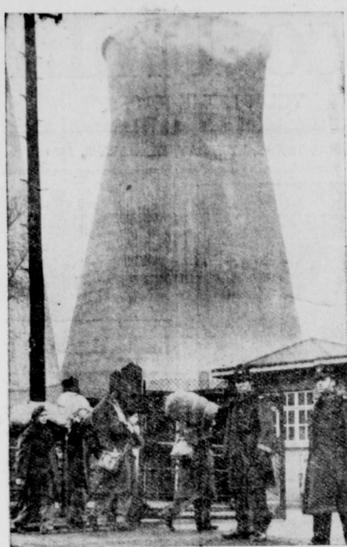
PREPARING FOR CRISIS—When a wildcat strike cut down the electricity supply in London, England, these troops moved into the Brimsdown power station at Enfield. They joined naval ratings who took over the work of about 600 strikers. More than 23 plants were involved.
