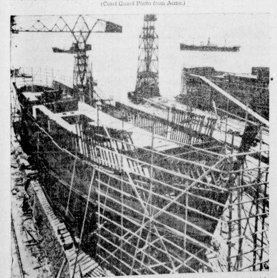
FOR DENMARK-This is a general view of a shipyard in Tamano, Japan, where three deadweight cargo ships, each weighing 5170 tons, are under construction for a Danish shipping firm. The first of the three to be launched is at the right background, the second is in foreground.
