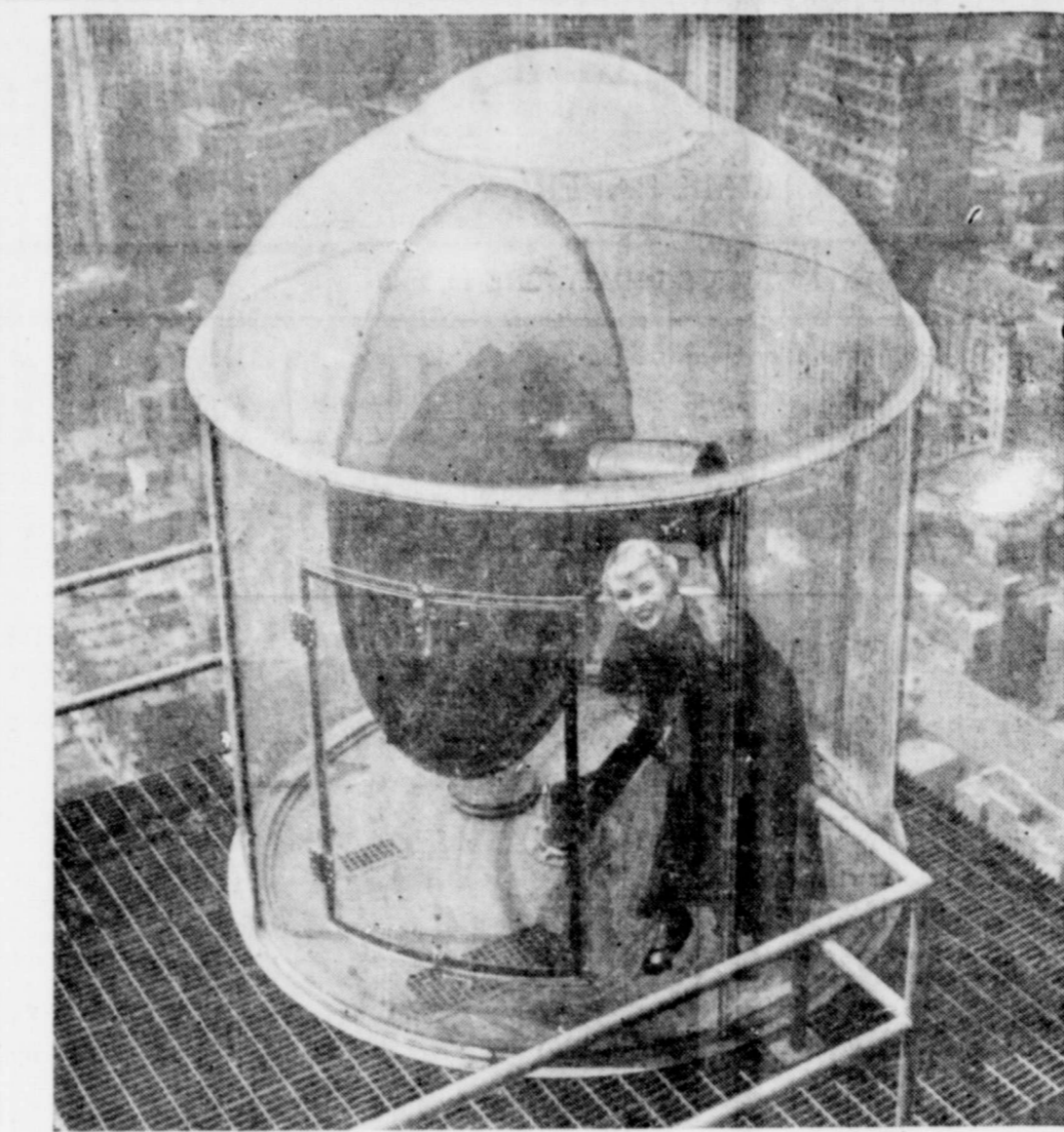
TOP STUFF —Kyle MacDonnell, pretty video star, inspects the latest plexiglass radome housing receiving equipment for television. Atop a New York skyscraper, Kyle investigates the "dish" which serves as a receiving antenna for remote television pick-ups.
