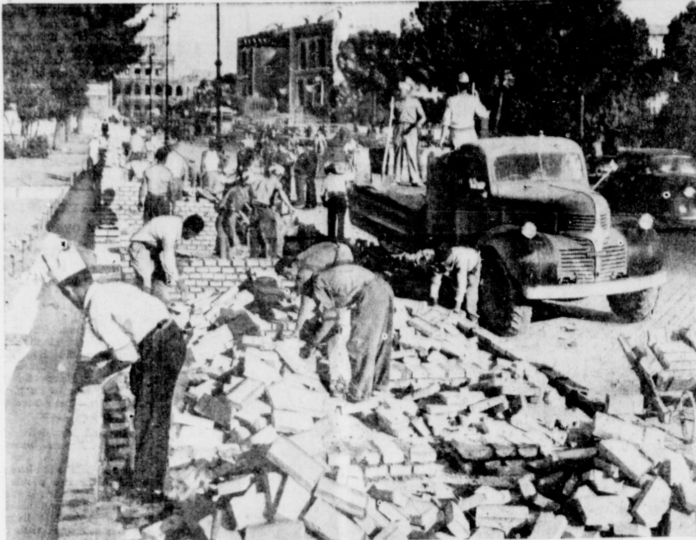
COSTLY REVIEWING STANDS—These workmen in Rome, Italy, are building brick ramps for the reviewing stands along Rome's Via Empiro. They were used for a military parade which celebrated the establishment of the Republic of Italy. Costly in money and labor, the construction took place along both sides of the street and was scheduled to be torn down the day after the parade. (Acme Photo by Albert Blasetti, Staff Correspondent.)
