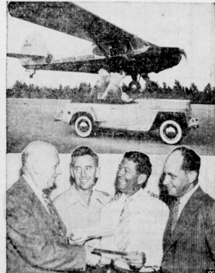
* Twice a day for six weeks, Bill Barris and Dick Riedel of Fullerton, Calif., repeated this stunt of refueling their Aeronca at 75 miles per hour. Their record-breaking endurance flight of 1,008 hours, 2 minutes, covered 75,000 air miles, the equivalent of three times around the earth. In lower photo, B. F. Tobin, Jr. presents the former military pilots with checks in behalf of Continental Motors, one of whose stock C145 engines kept the plane aloft by running six weeks without a "miss". The others, left to right: Riedel, Barris, and Don Young, aviation engineer for MacMillan Petroleum Corp., whose Ring-Free motor oil was used throughout the flight.
