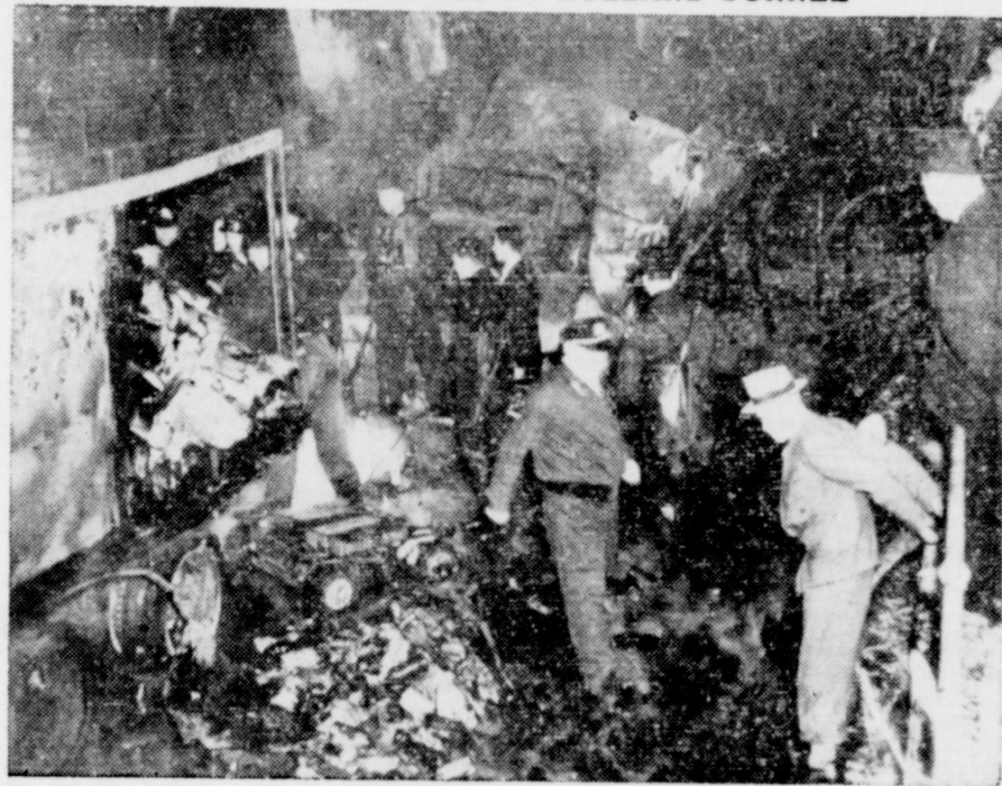
Police and firemen examine debris of burned trucks in the blasted Holland Tunnel after a chemical truck caught fire, exploded, and set other trucks on fire. Several police and firemen were injured fighting the fire and a dock worker was overcome by smoke and fumes.
