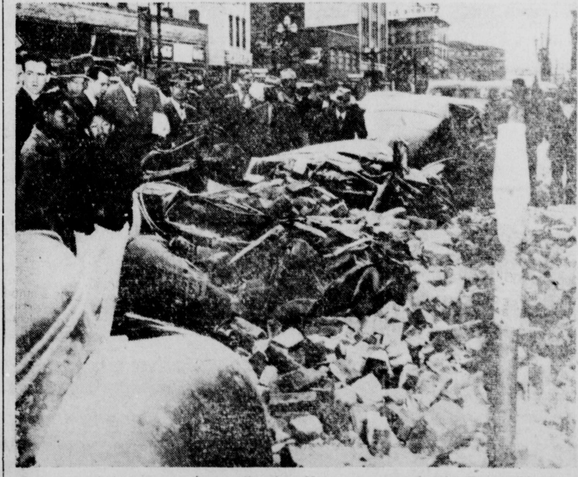
Curious crowds inspect a parked automobile in downtown Seattle, Oregon, following a severe earthquake. Many automobiles were demolished by falling bricks from buildings which were cracked by the earth's movements. — ACME.
