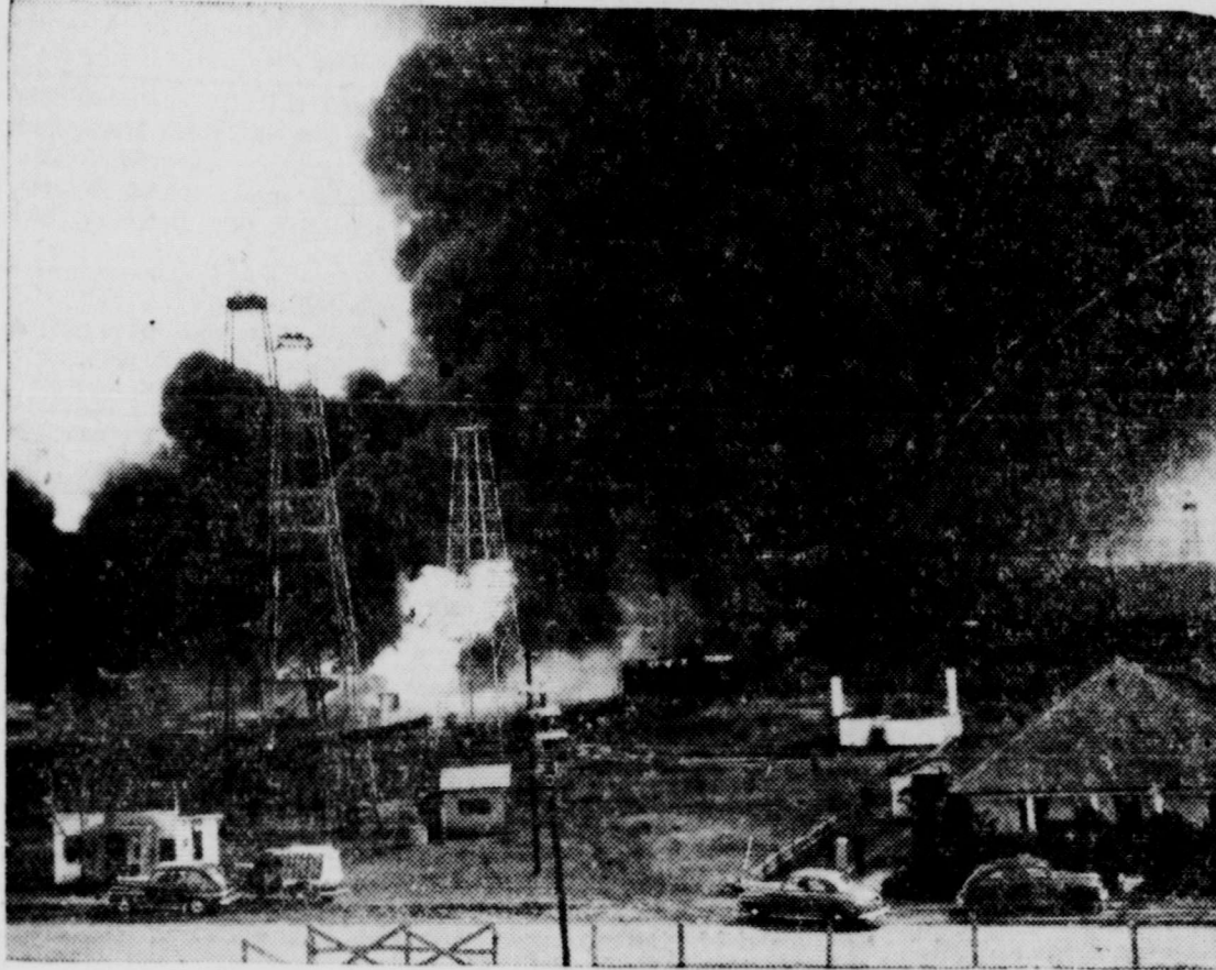
Fire sweeps through the Warwick Wax Co. in Kilgore, Texas. The fire started in a trash blaze and spread to a small tank arm. The tanks burned furiously for several hours, destroying telephone lines and disrupting rail traffic. — NEA.
