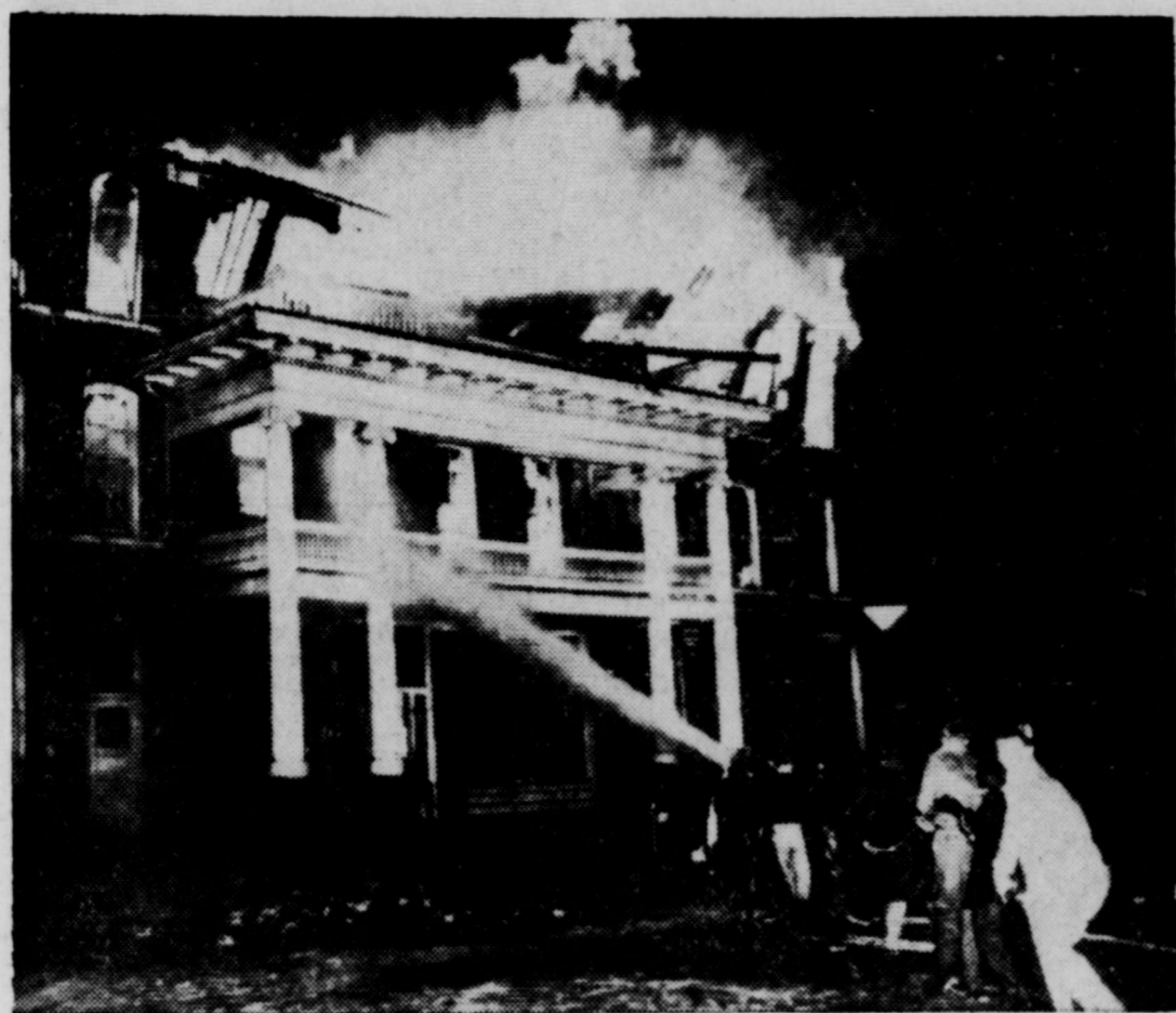
Walls of the 75-year-old Grand View Hotel in Ripon, Wisconsin, crumble during a fire which destroyed the building. Authorities feared at least five persons died in the blaze. Most of the hotel's 48 guests escaped to the street in their night clothes—ACME.
