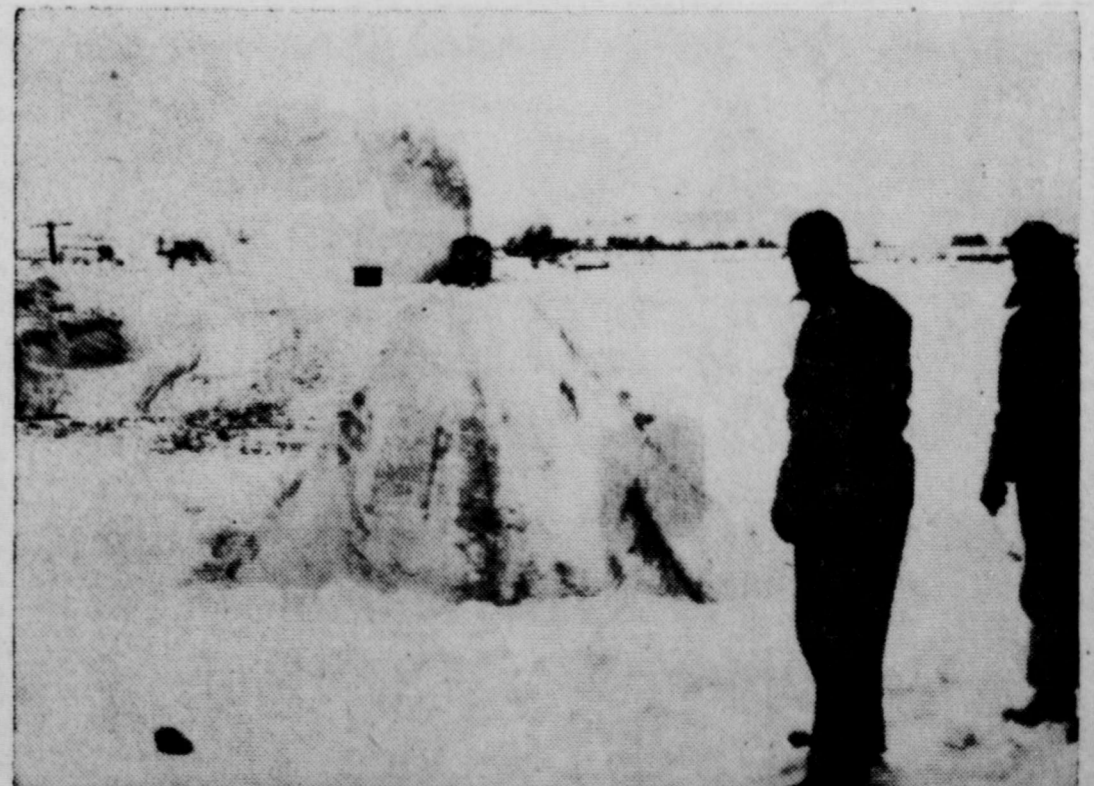
At Belmont, near Alliance, Nebraska, a Burlington Railway rotary plow backs up for another run at 15 to 20 foot snow drifts in an effort to clear the tracks. The plow, using its own power plus two steam engines, hits the drifts, then backed up for a new whack. Shoveling crews in foreground stand on packed drifts to scoop snow into the rotary when drifts are above 15 feet—ACME.
