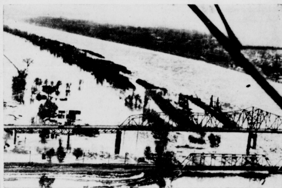
An airview of the ice choked Missouri River at Atchison, Kan., showing the railroad and highway bridges over the river and flooded lowlands. Held back by huge ice jams, the river has forced evacuation of homes along both the Missouri and Kansas banks. The main channel of the river is plainly visible.
