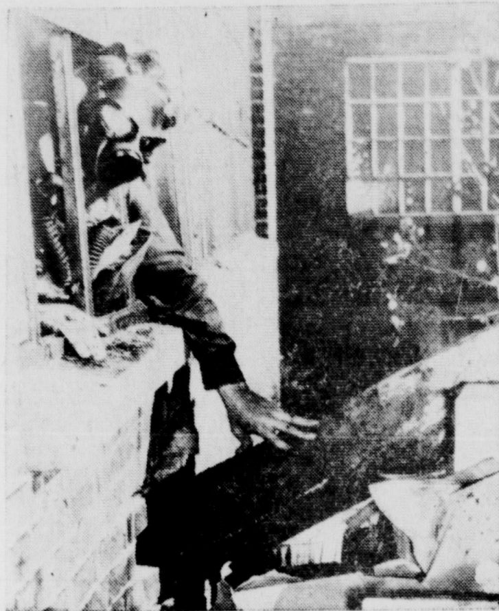
Three employees were injured when an ammonia tank exploded in the basement of the Fasano Pie Company in Chicago. Nick Loschetter, Chicago fireman, points to large pipe that was driven through a three foot wall when the explosion occurred.—(NEA Photo).
