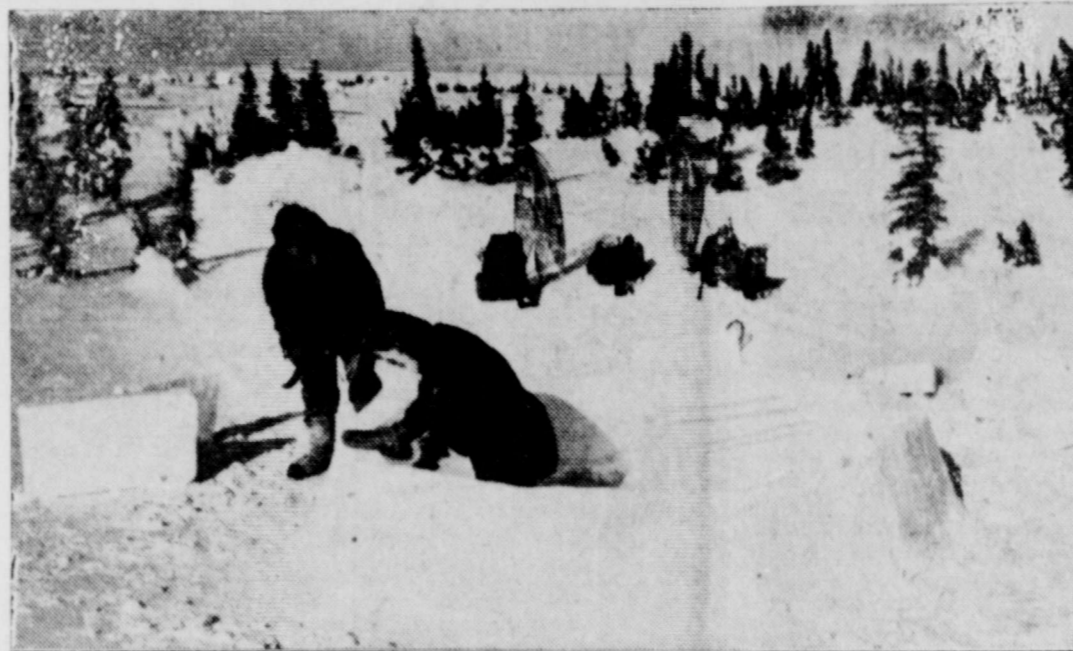
AMERICAN SOLDIERS BUILD SNOW HUTS—The U. S. Arctic Infantry Patrol erects an igloo in the extreme northland. The snow in the lee of trees or rocky obstructions is too soft to be used in igloo building but packed snow in open drifts is ideal for this purpose. With the base circle complete, the men "chink" loose snow into seams, and shave the surface rim at an angle to start a second row of blocks canted inward. These "snow masons" have completed the first section.
