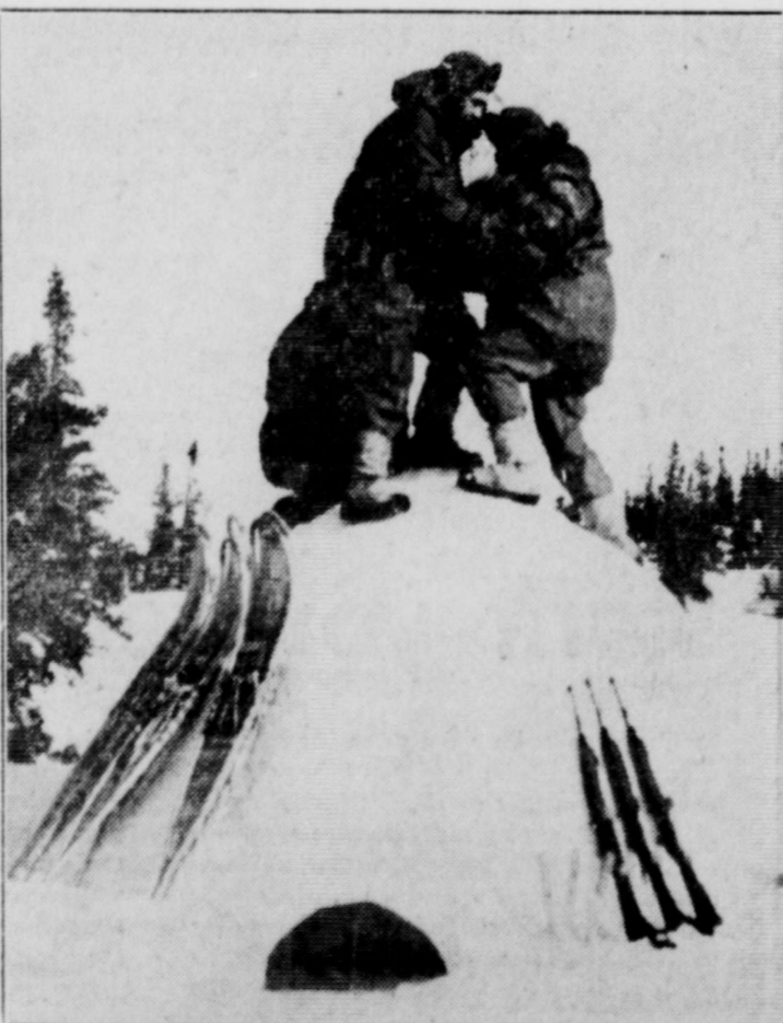
TESTING THE ROOF OF AN IGLOO—These soldiers of the U. S. Arctic Infantry patrol have completed a snow hut on the shores away up north and are making sure that the dome will withstand more than 500 pounds weight. These huts provide shelter for troops for many weeks.
