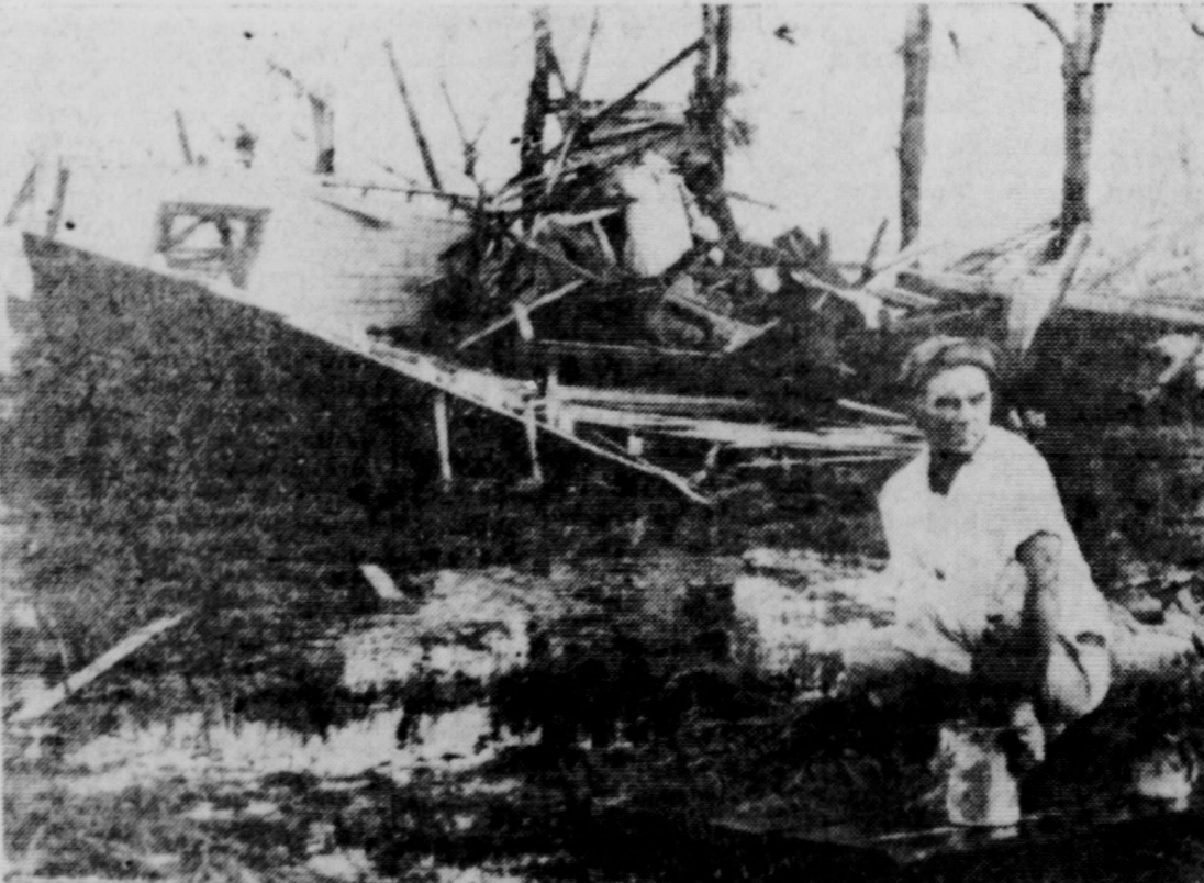
Bill Fernandez sits before his tornado battered home after winds flattened it during the hurricane which swept over southern Florida. Flood waters in the background cover the ground where the house foundation stood. Fernandez lost all his possessions at his Opa Locka, Florida home.—(NEA Telephoto).
