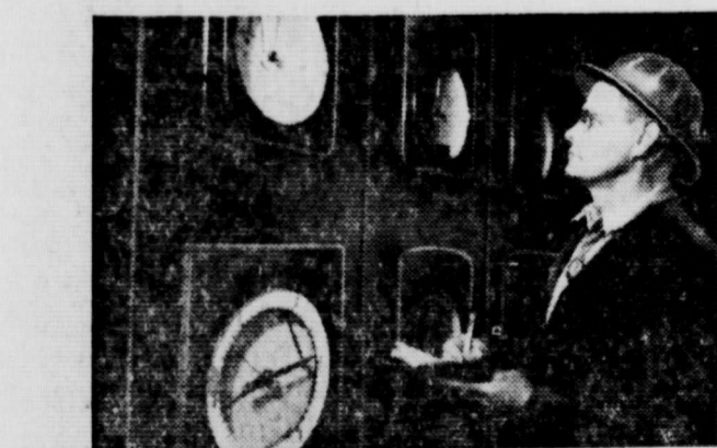
THE INDUSTRY IS EXPANDING ITS REFINING CAPACITY to meet your demand for finished petroleum products, and to increase the output of existing facilities. In 1947, Humble refineries increased their output by 12%. This picture shows the control panel at one of Baytown refinery's two catalytic cracking units; these units enable the refinery to get more finished products from each barrel of crude oil.
