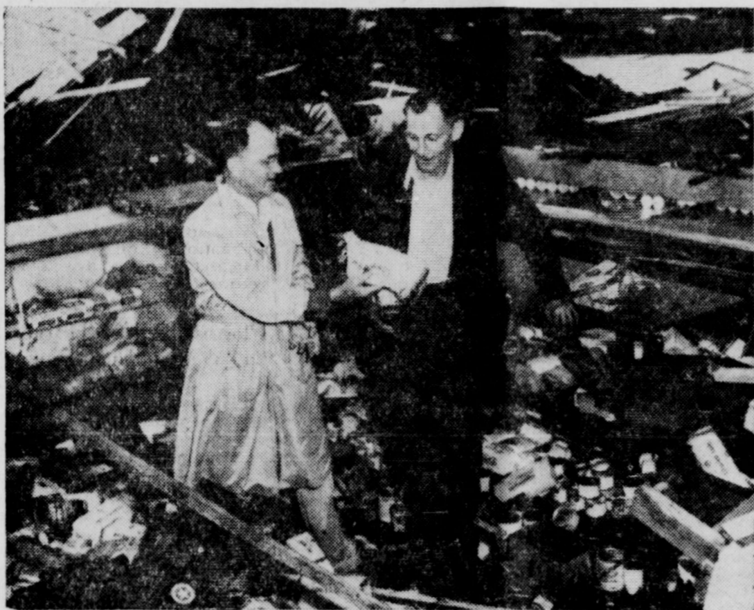
E. B. Bennet, left, and L. E. Blaylock salvage a few groceries from their McKinney, Texas, store after a tornado had completely destroyed the building. The tornado struck suddenly and damaged the community to the extent of three million dollars. Fortunately only three persons lost their lives in the disaster. (NEA Telephoto).
