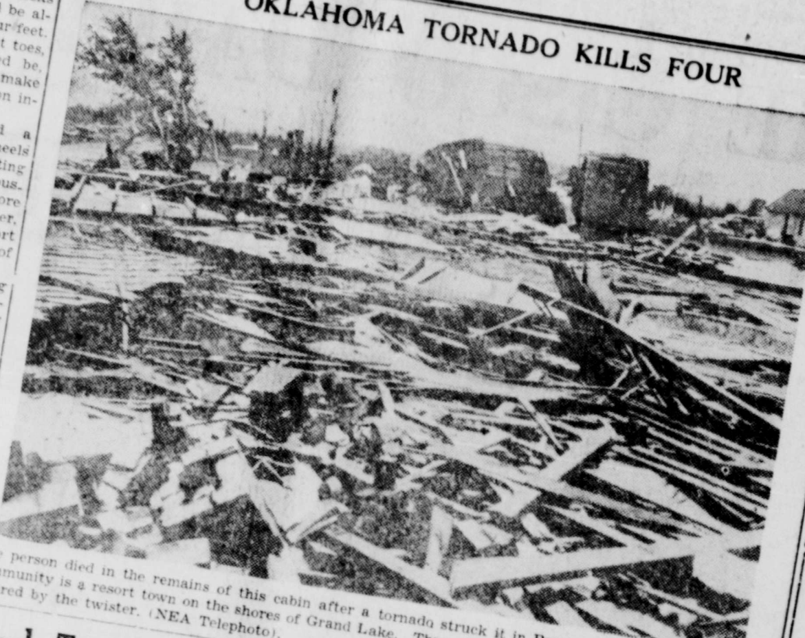
One person died in the remains of this cabin after a tornado struck it in Bernice, Oklahoma. Three other persons were killed and forty were injured by the twister. (NEA Telephoto).
