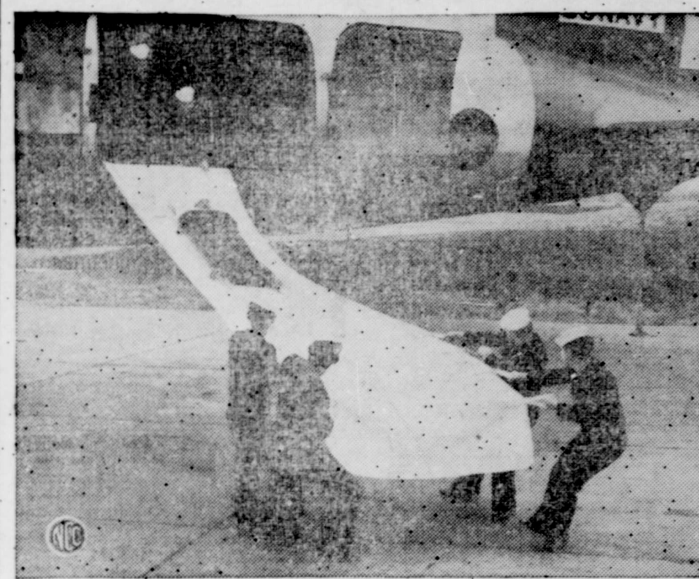
After a crash landing, Navy litter patients can be slid to safety down a strip of heavy duck canvas. Now carried aboard all VR-3 evacuation aircraft, one end of a 26 x 3 1/2 foot canvas strip is hooked to floor rings near the cargo door. Two or more crewmen hold the other end tautly away from the airplane while other crewmen gently slide the litter patients down from the nine-foot height. (U. S. Navy photo)
