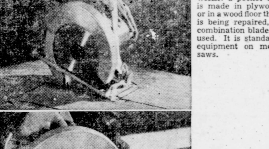
WHEN a pocket cut is made in plywood or in a wood floor that is being repaired, a combination blade is used. It is standard equipment on most saws.
