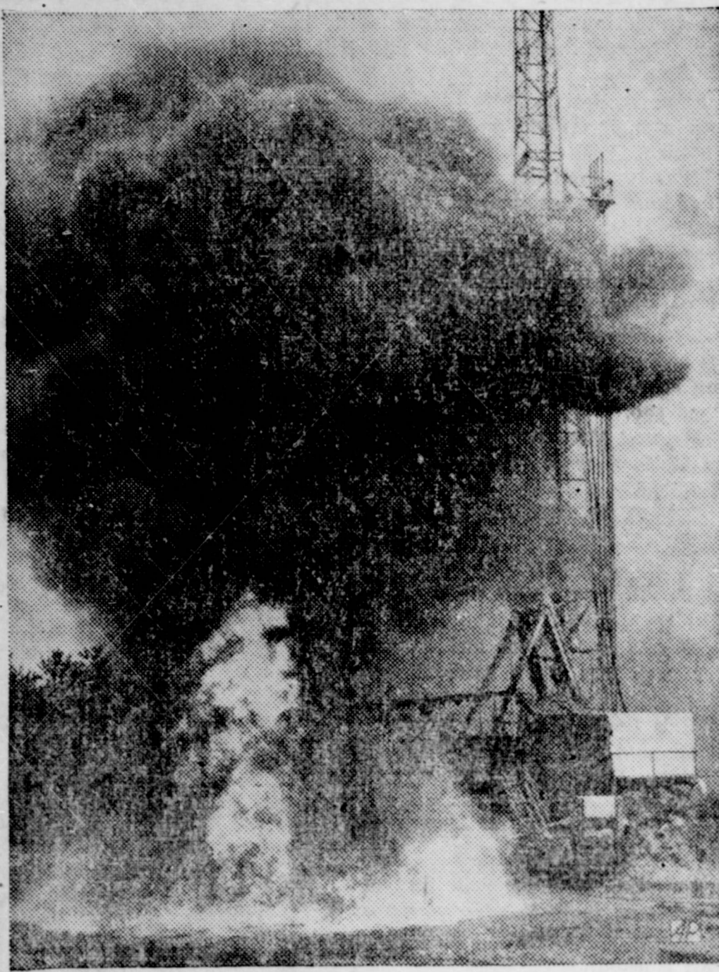
The oil discovery well was brought in six and one-half miles north of Marshall in the northern part of the Woodlawn oil and gas field. It produced 22.5 barrels an hour of 41.3 gravity crude. It was perforated in the Pettit lime at 6,467-77 feet. The fire in the foreground is slag oil burning in the slush pit. (AP Photo).
