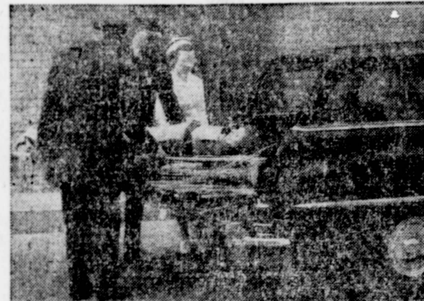
Here a patient is rolled quickly into a secure and comfortable position inside the ambulance, where a nurse may be seen sitting in the attendant's position, ready for the quick run to the hospital. When not in use, the collapsible cot folds away behind the rear seat.
