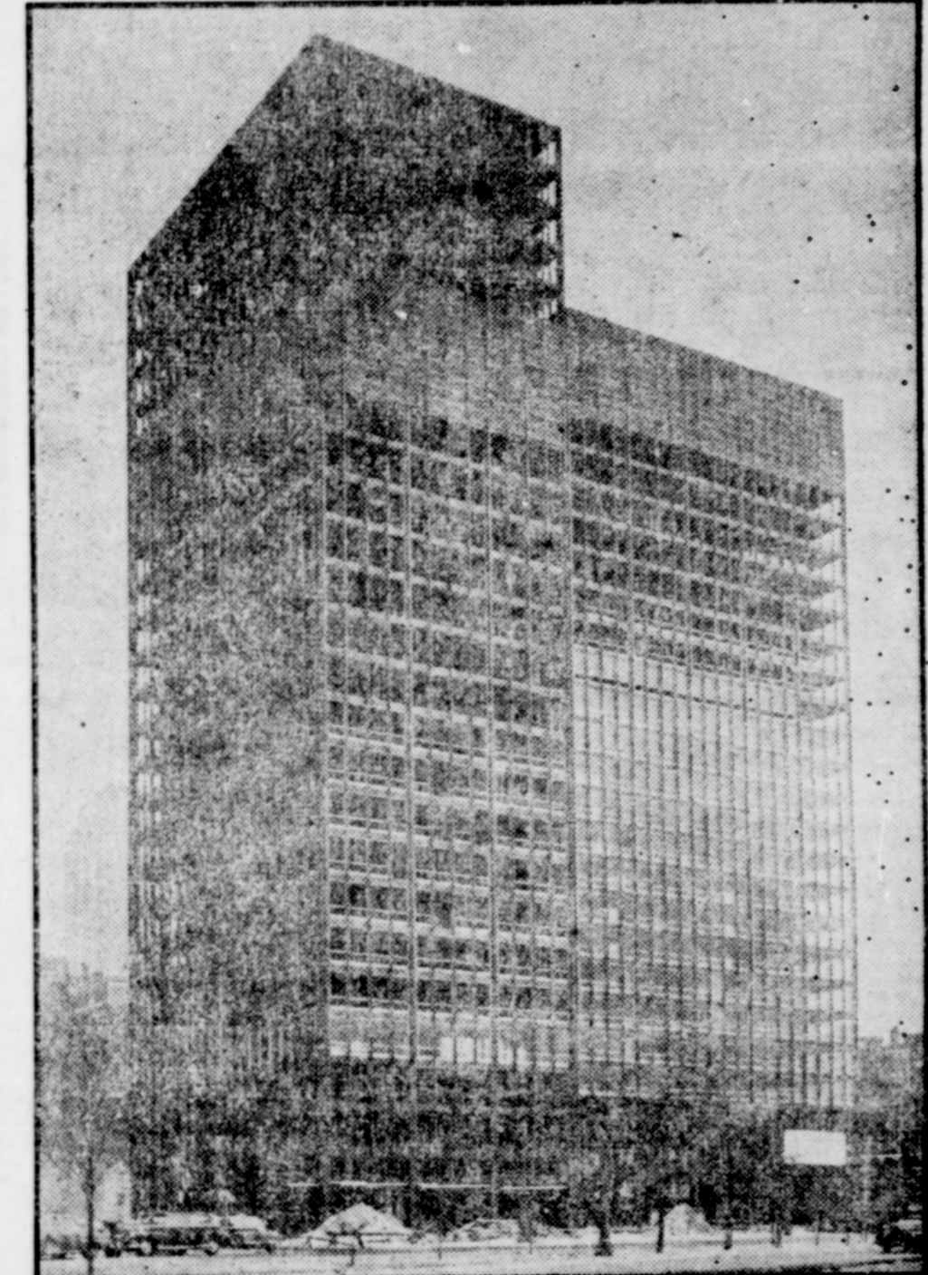
PEOPLE IN GLASS HOUSES —The entire outside of this 26-story apartment building in Chicago is made of steel and glass. When completed, the structure on Chicago's Lake Shore Drive will have more glass than the Merchandise Mart, which is the world's largest building. Two garages will be located in the basement and sub-basement of the "Glass House."
