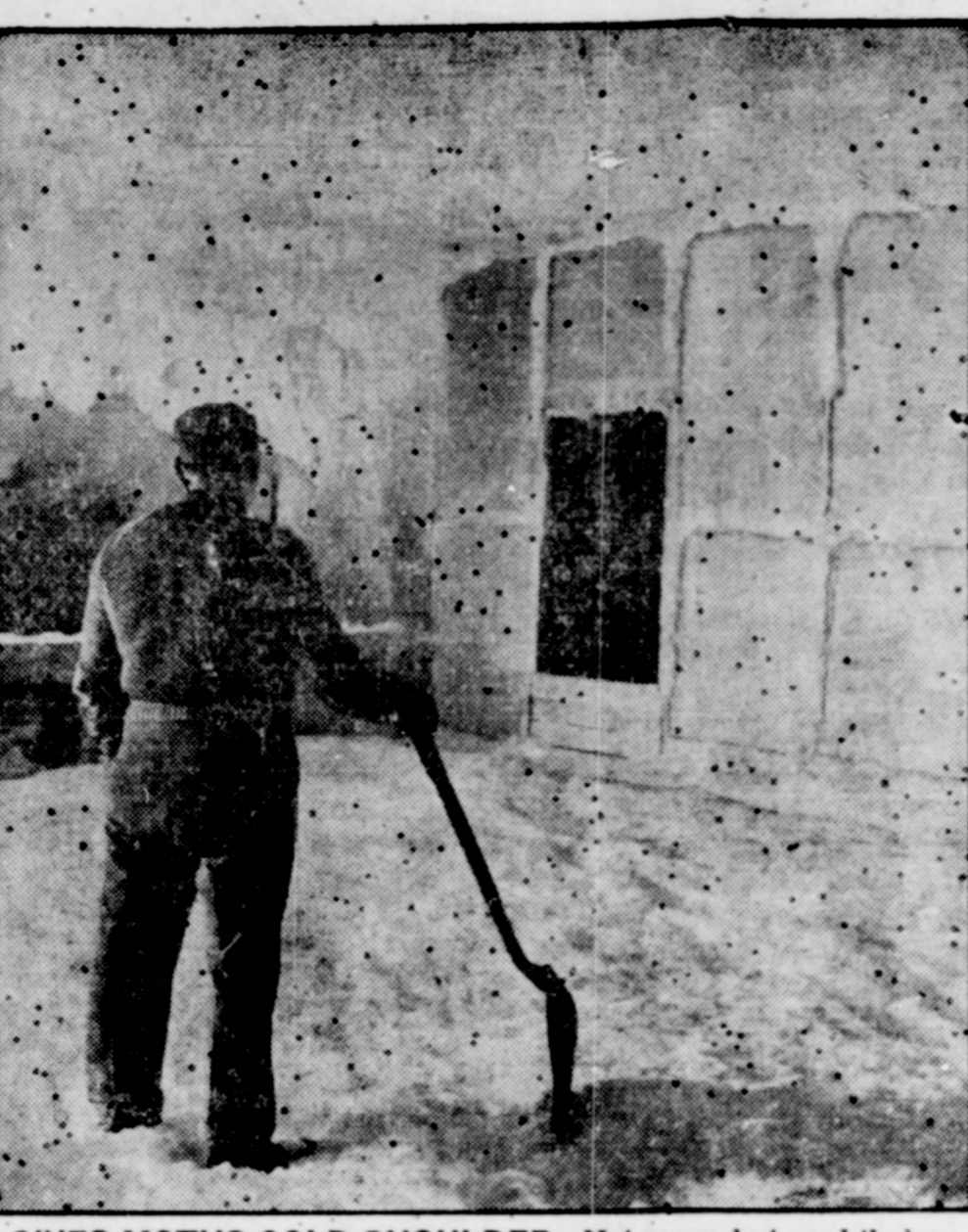
GIVES MOTHS COLD SHOULDER —Not snow, but naphthalene flakes line the walls and ceiling of this subliming room at a plant in Kearny, N. J. The flakes, used in the manufacture of moth repellents, are produced by evaporation and condensation of liquid naphthalene, which is extracted from coal. The "snow" covering is shoveled from this room for further processing.
