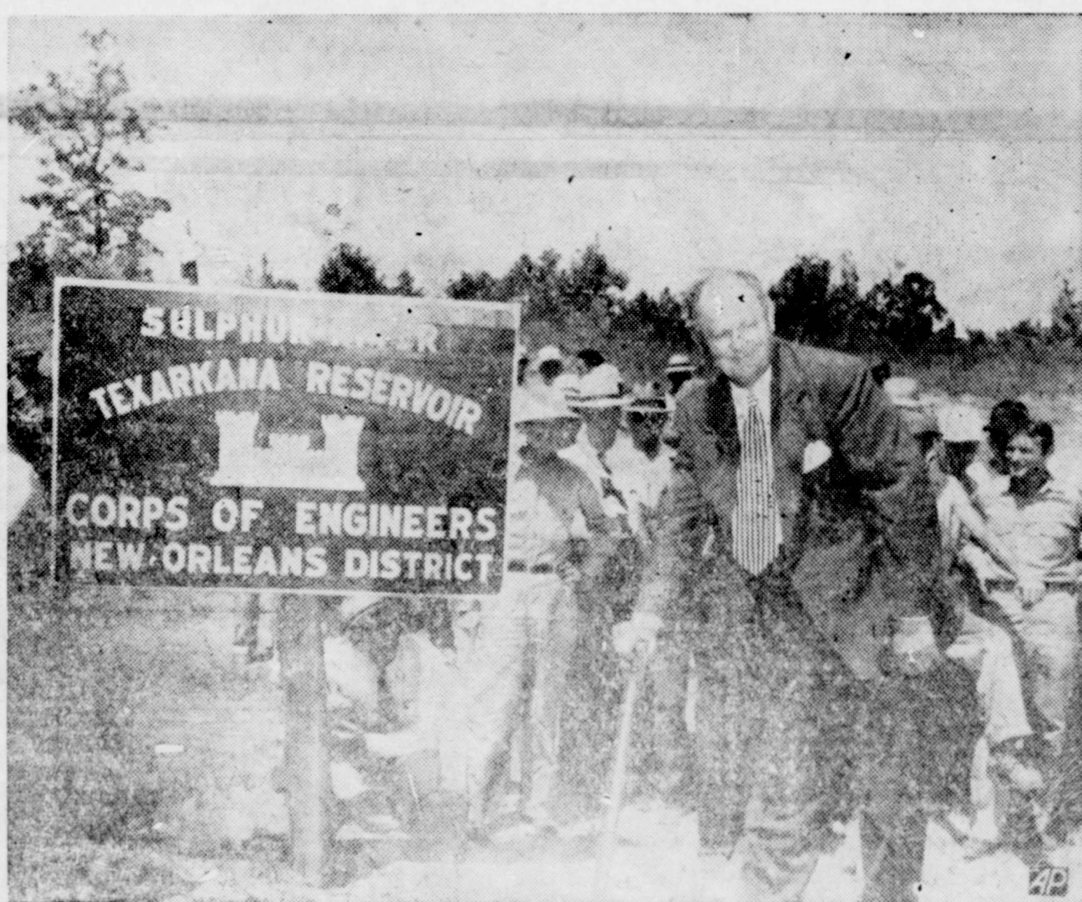
GROUND BREAKING FOR NEW DAM — Congressman Wright Patman breaks ground on the site of a $26,000,000 flood control project on the sulphur river 11 miles south of Texarkana, Texas. The dam, one of five in the red river basin below Denison Dam, "is a new industrial area for East Texas," said Patman. (AP Photo).
