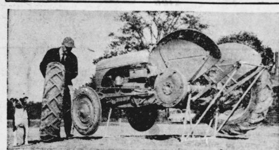
The self-lifting tractor is now a reality. It rises any height, up to four inches, virtually drawing itself up "by its own bootstraps." The lifting operation is accomplished by placing light tubular frames beneath the axles, connecting the rear to the two arms of a Ford-Ferguson tractor's hydraulic linkage and lightly touching the "fingertip control" lever which is one feature of the Ferguson System. The entire operation takes less than one minute.
