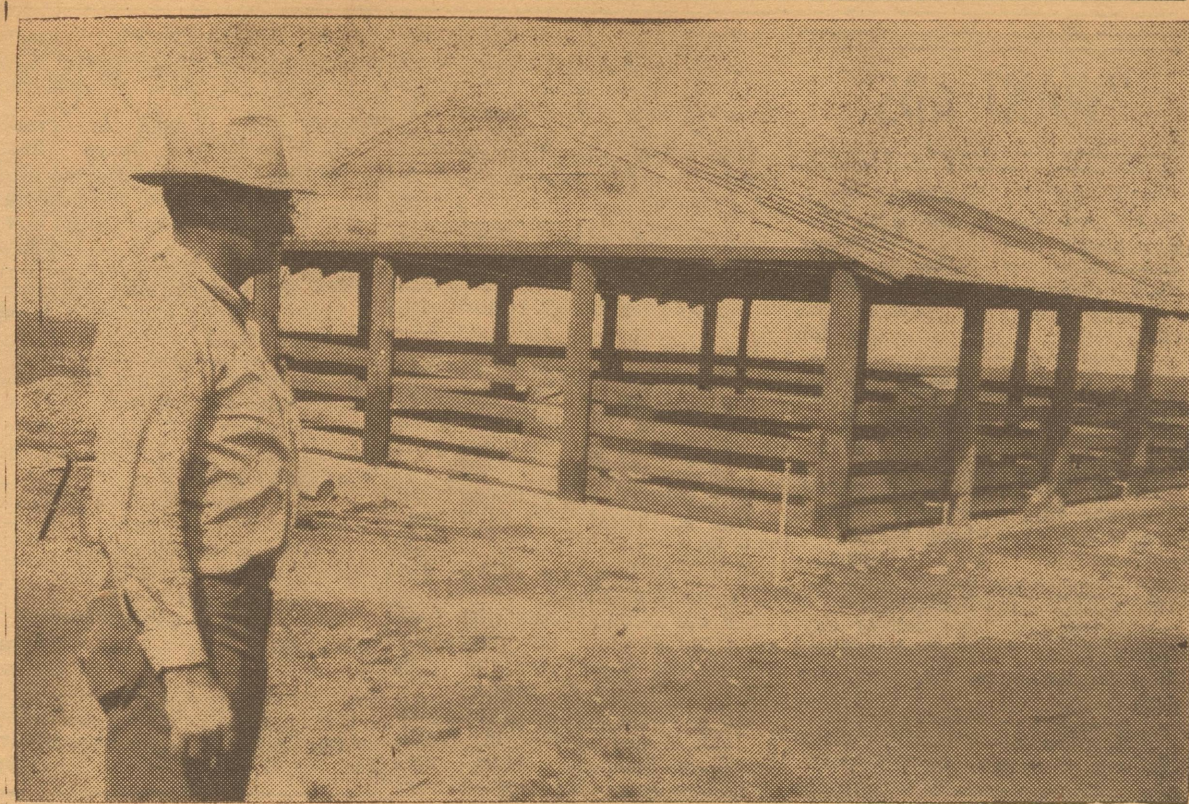
FANCY PIGHOUSE — Doyle Cummings shows what a modern-day "pig parlor" looks like from the outside. The open construction provides good ventilation, yet the pigs are protected from the weather.
