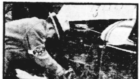
The official sealing of crankcases after fill of five quarts was out in. No addition of oil was permitted in this "destruction" test.
