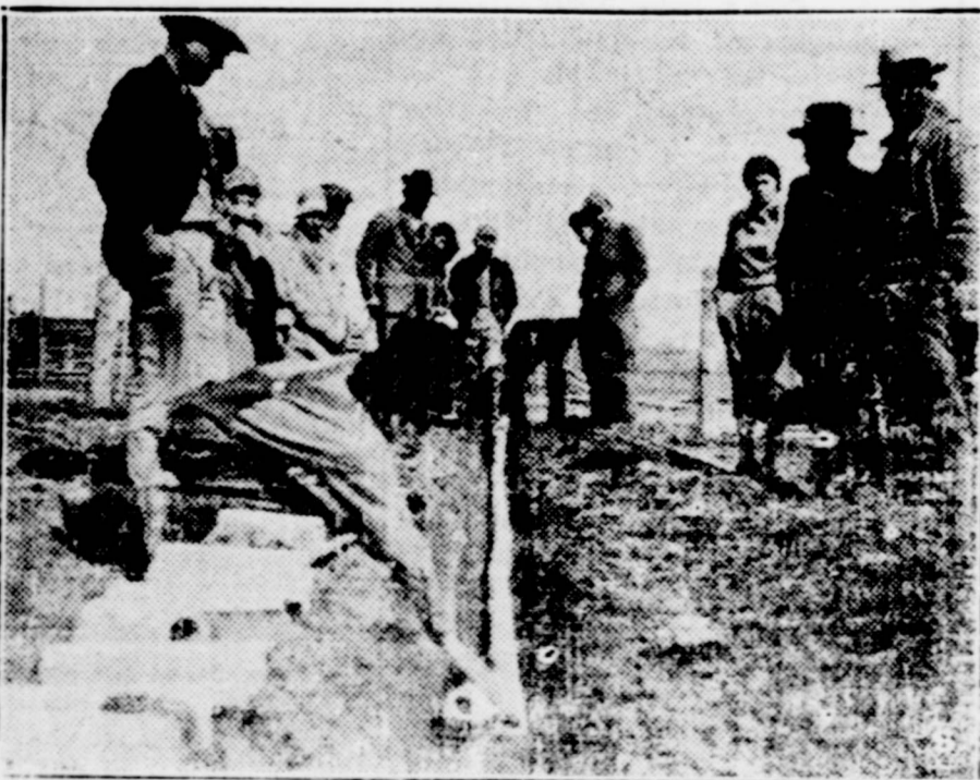
Here is shown a sub-irrigation installation in Grayson county, Texas, by B. F. Gray on the Hart farm. Sub-irrigating gardens using lat's tile costing about one cent a foot is one of the big developments in gardening in Texas. The move is so strong this year that many are making cheap concrete tiles at home for the purpose.
