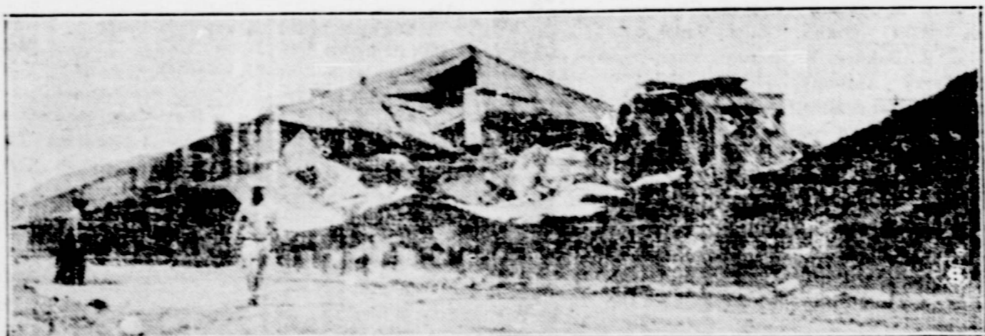
Damage approximating $125,000 and injury to three employees resulted last week when fire destroyed the plant of the Texas Eth Carbon company near Pampa, Texas. The three men injured were overcome by heat and fumes and taken to a Pampa hospital. Fire destroyed 600,000 pounds of carbon black and endangered 25,000,000 pounds stored nearby.
