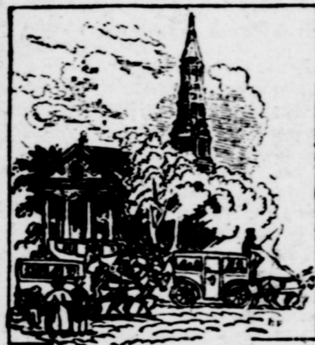
St. Paul's Chapel, Broadway, Fulton and Vesey Streets, the Oldest Church Structure in Manhattan.
