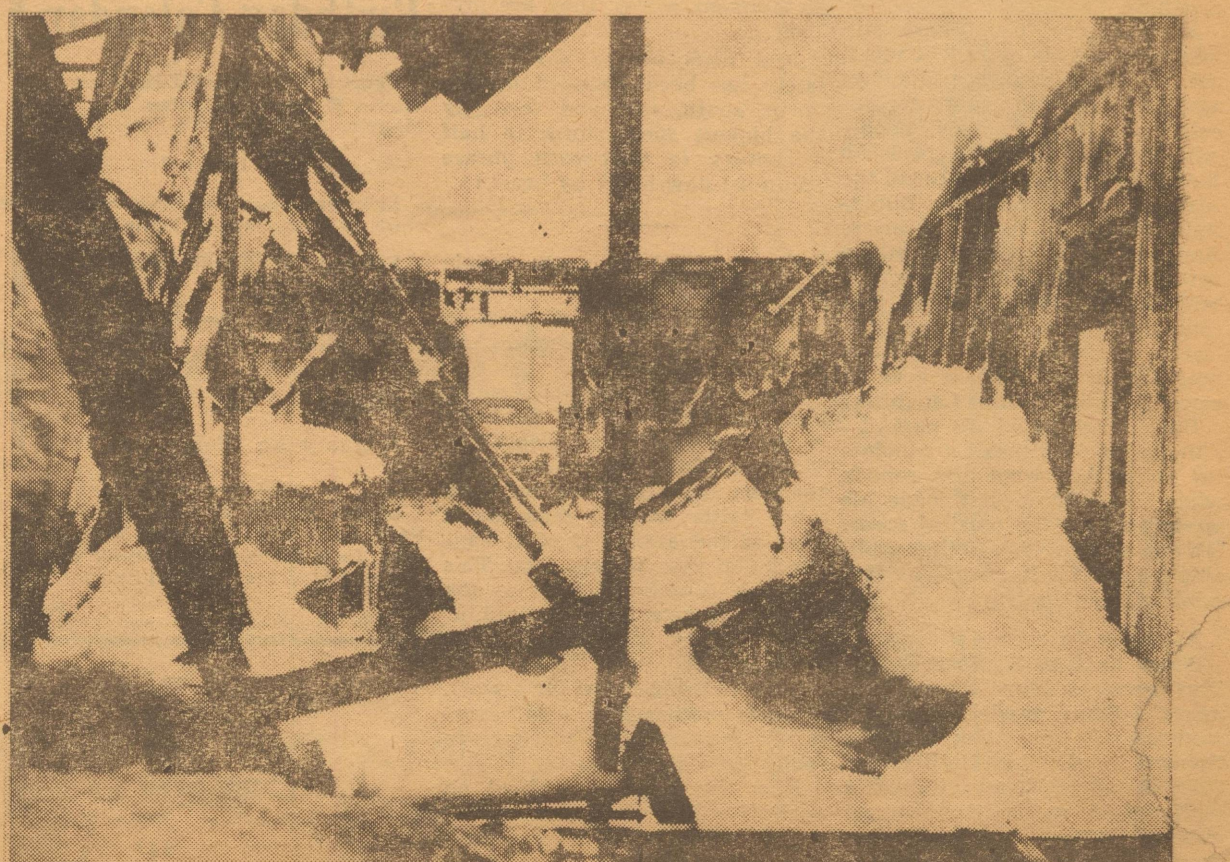
Fire still smoldered in the Friona Locker Plant one long cold week after the flames broke out. Members of Friona's Volunteer Fire Department left one hose running on insulation which continued to burn. Snow piled high on the blackened ruins and left this graphic contrast. Star Photo
