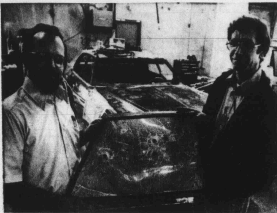
THEY MAKE ARMORED SEDANS — Fred Mueller, left, and Ron Chandler, vice presidents of Tetradyne Corp., in Richardson, display a bullet proof window that had been tested and shown to resist high-powered rifle shots. A window of this type will be put in the sedan in the background along with armor plating to protect the occupants for up to a minute of an attack as long as bazookas and armor-piercing bullets are not used.
