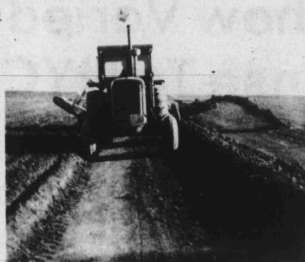
TERRACING MACHINE Completing Part of Half Million Feet of Terracing
