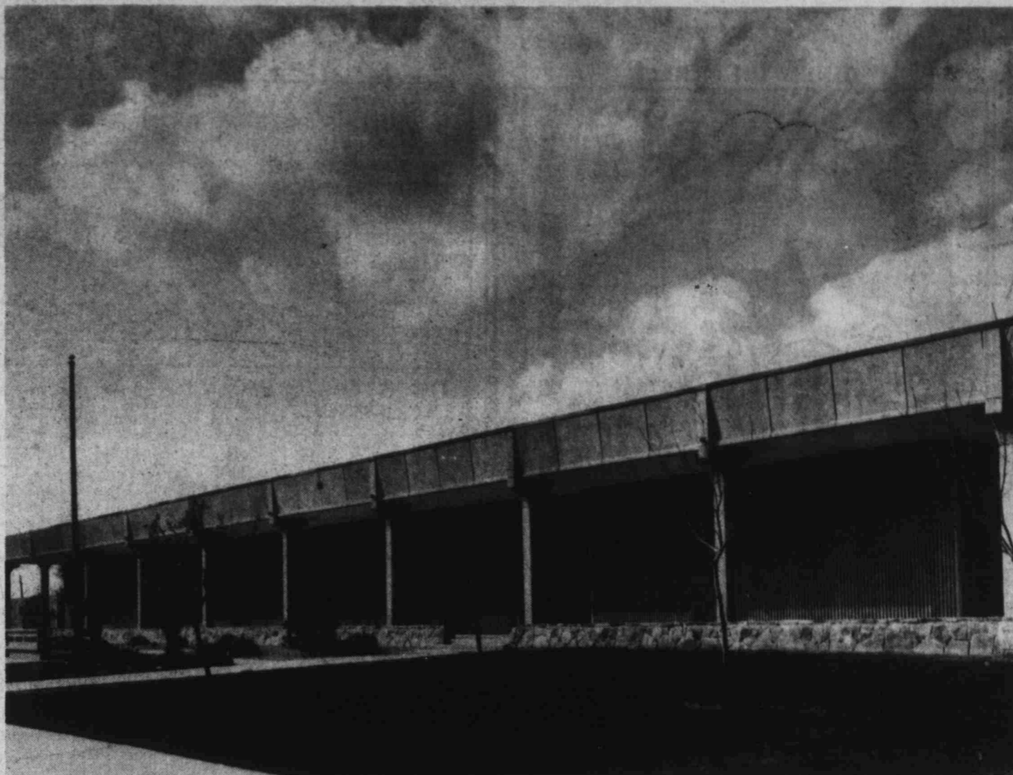
OPEN HOUSE SATURDAY — The New Martin County Courthouse will be dedicated in ceremonies at 3 p.m. Saturday with District Judge Ralph Caton giving the welcome followed by a two-hour open house. The event is hosted by Martin County officials and the public is invited.
