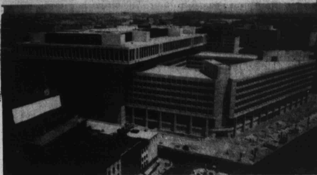
FBI HEADQUARTERS — The new headquarters of the Federal Bureau of Investigation, named the J. Edgar Hoover Building is pictured in this view looking northeast. Pennsylvania Avenue is visible in the lower right corner of photograph. The $128 million structure is slated for formal dedication Tuesday in Washington.
