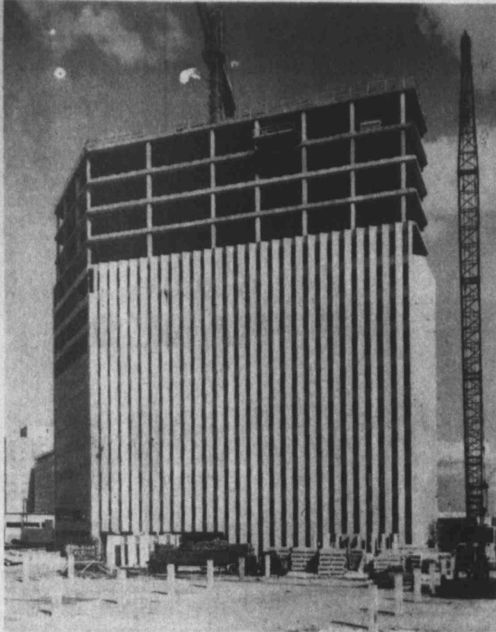
TOPPED OUT —The Midland National Bank Tower, a 14-story, 230,000 square foot joint venture project between Midland National Bank and Gerald D. Hines Interests, Houston, topped out Aug. 14, reaching its full height of 203 feet. Installation of precast panels is currently under way with completion slated for September. Commencement of tenant work began in mid-August and occupancy of the new tower is planned for this fall.
