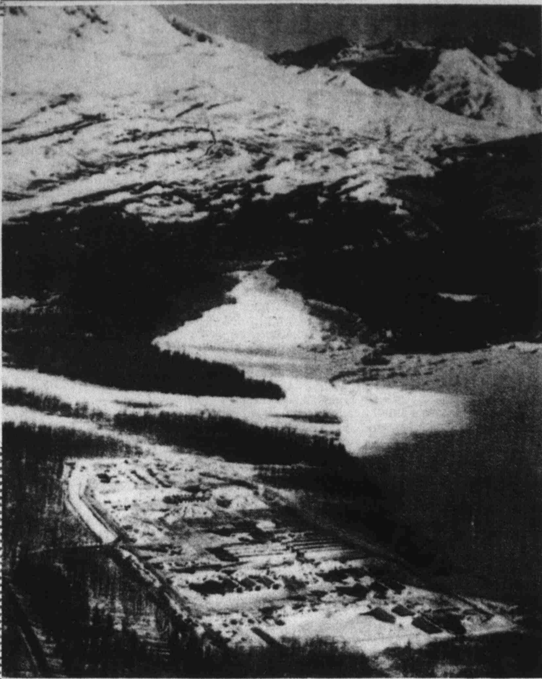
SCENIC CAMP — Sheep Creek Camp, one of 20 pipeline construction camps on the trans Alaskan pipeline project, is located about 20 miles north of Valdez, Alaska. The camp will have a bed capacity during 1975 to accommodate 1,008 workers. The start of Thompson Pass is shown at the top of the photograph.
