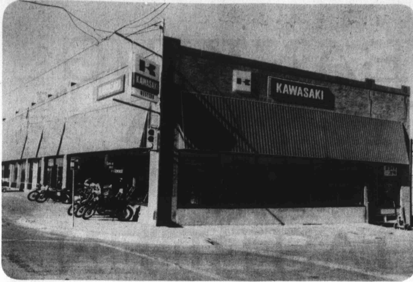
DOWNTOWN HALF BLOCK REFURBISHED — The Homan building, located at Third and Scurry Streets in downtown Big Spring, was given a major face lifting before it was occupied by the Western Kawasaki motorcycle firm. It was opened during 1974. (Photo By Danny Valdes)
