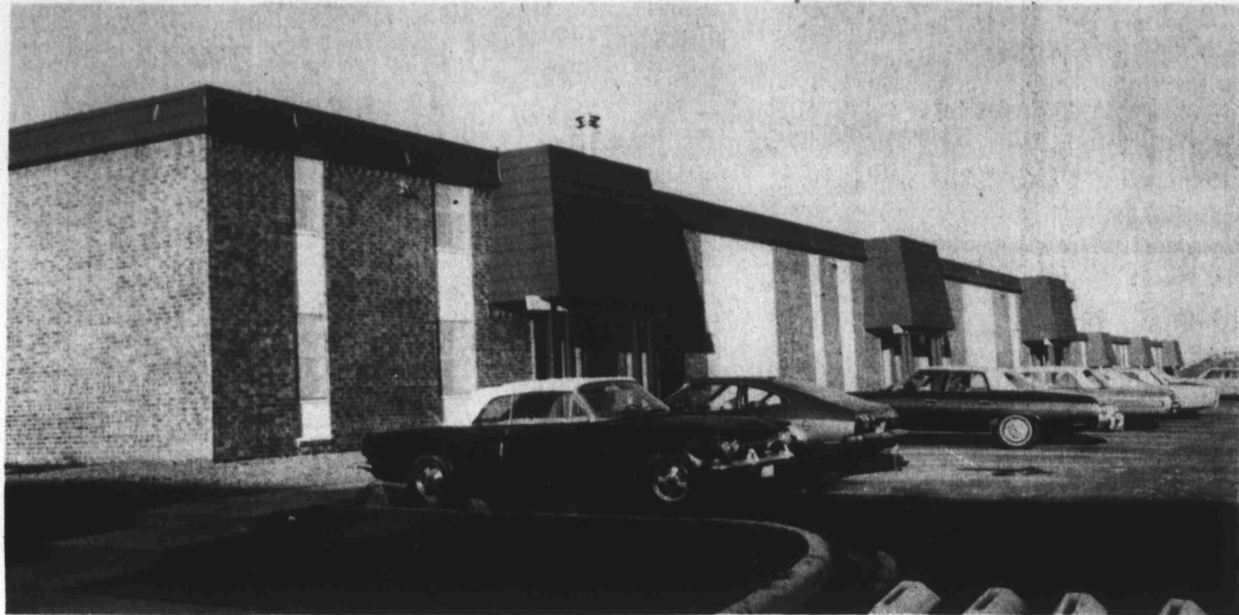
HELPED EASE A PROBLEM — The park Village apartment complex, located near Marcy School in the Douglass addition, helped ease a serious housing shortage in Big Spring when its first units were opened last year. Winston Wrinkle and Bill Sheppard are the two local men who developed the complex.
