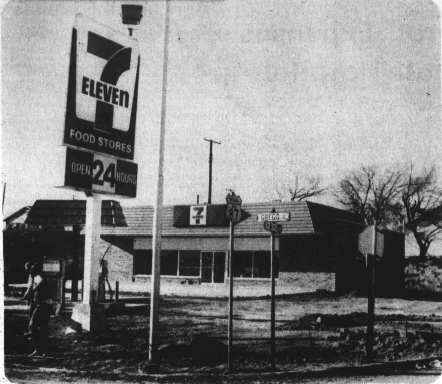
FINISHING TOUCHES — When 1974 drew to a close, construction on this 7-11 Food Store, located at 8th and Gregg Streets, was nearing an end. The structure helped swell Big Spring's building permits to a record high. (Photo by Danny Valdes)
