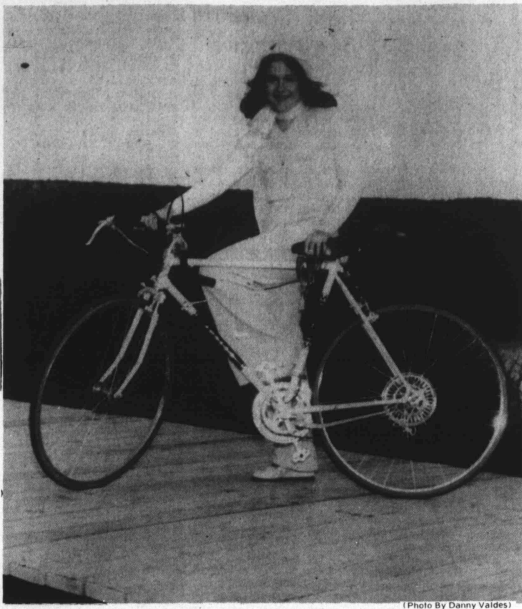
BIKING ON NEW TRAIL — Miss Debora Brown, a Big Spring High School junior, pauses on a new bridge over the "hike and bike" trail. The city was building the bridges this week, as the last part of the trail construction job. Starting by Whipkey Road, the trail runs by the Cosden Lake, through brush, by the Big Spring and over to Comanche Trail Park.
