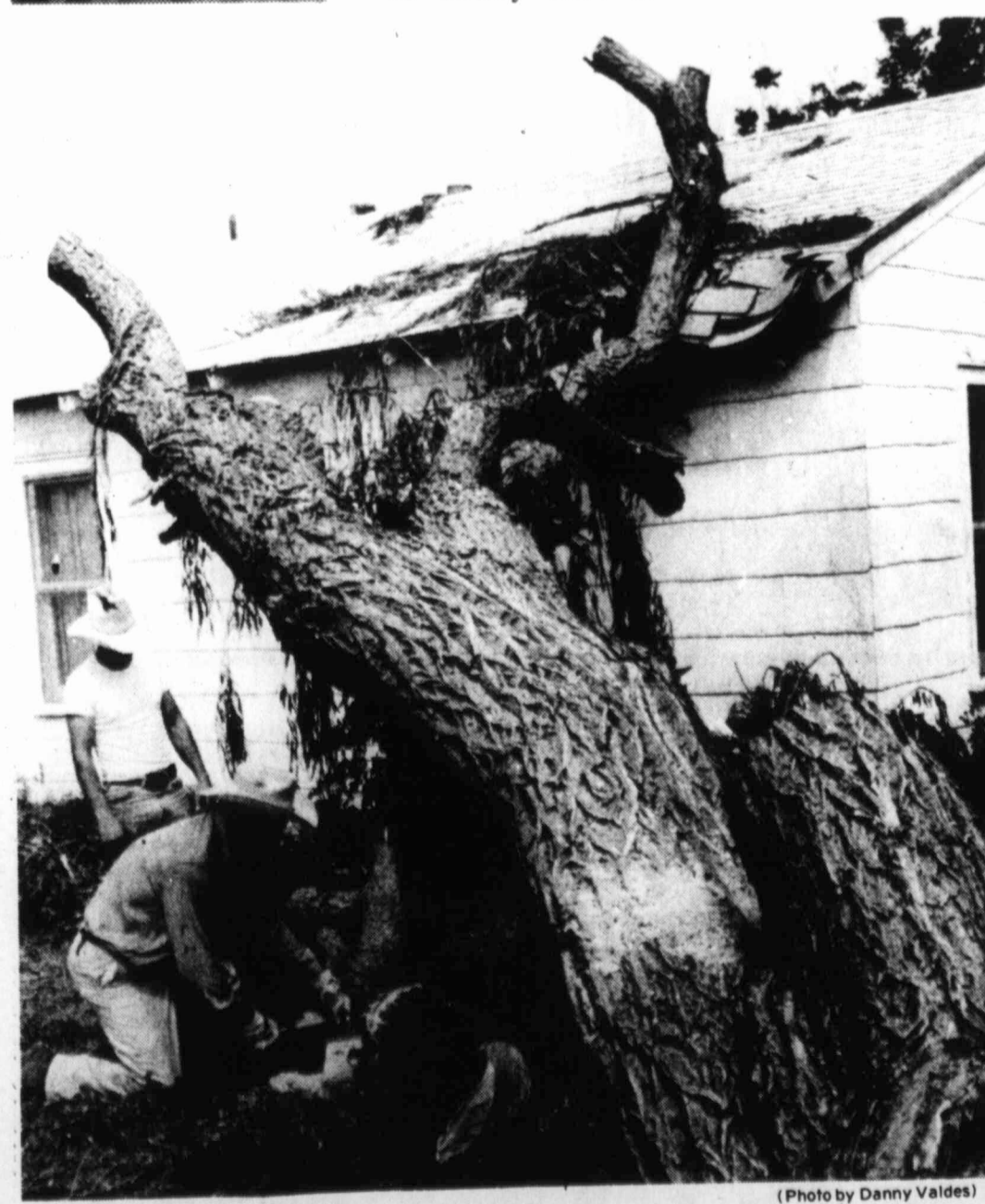
AN OLD FRIEND, DEARLY DEPARTED — A 25-year-old willow tree in the yard of Ella Moore, 2410 Scurry Street, was uprooted by the vicious winds which struck parts of the city Saturday evening. A section of the roof of the Moore home was damaged when the tree fell. Workmen here saw the tree limbs in order to help in its removal.
