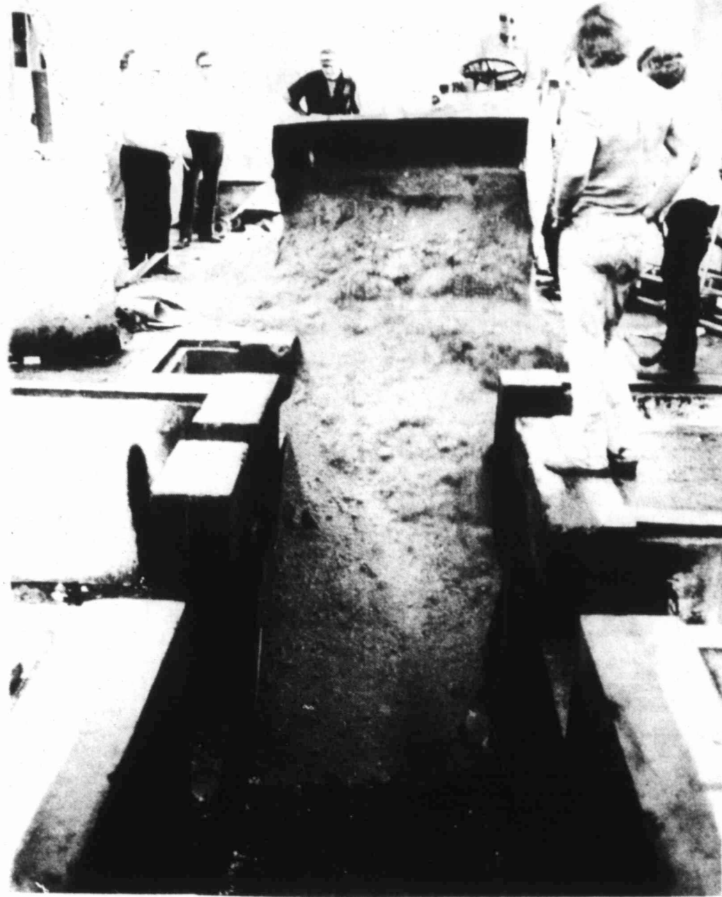
GAPING HOLE FILLED —The hole in The Herald's back shop which once contained the old letterhead press is filled with dirt before the area is smoothed over with concrete and converted into a storage area. The new Goss Community press which the newspaper is now using is located in the rear south portion of the building.
