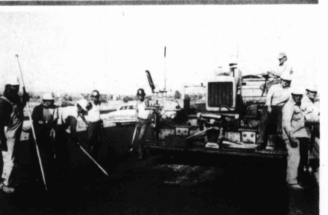
TEMPERATURES RISING — It was hot enough Tuesday for a person resting under the shade of a tree but for these highway workers stabilizing a segment of Interstate 20 east of town the temperatures were way up there. The chore calls for lots of patience and thick-soled shoes.
