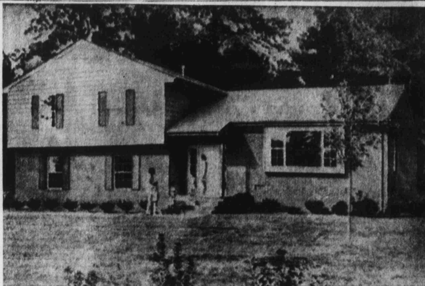
HOUSE THAT TRASH BUILT — This house in a suburban Richmond residential area was constructed entirely from recycled materials. The house contains aluminum scrap, crushed glass, recycled newspaper, fly ash, wood
