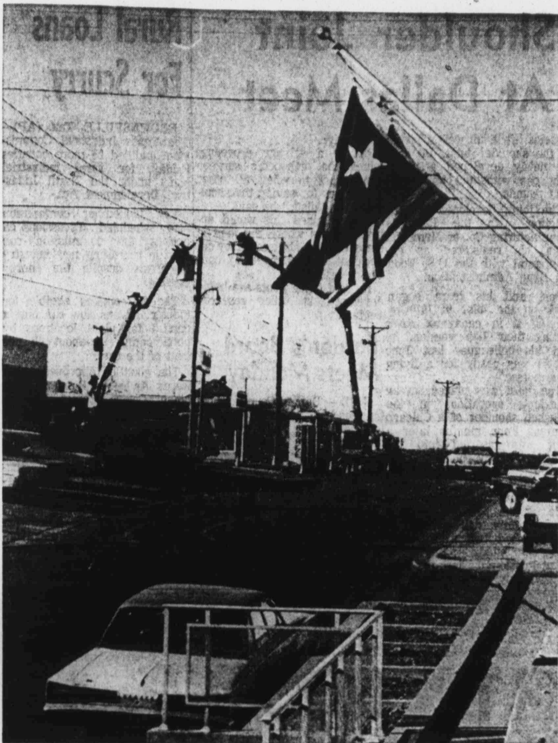
NEW POLES — Texas Electric Service Co. in Phase II of replacing poles on Gregg Street from wooden to steel for more efficiency and a modern look, according to Tom Locke, division manager.
