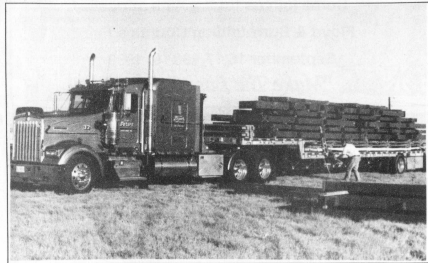
UNLOADING THE STEEL FOR UNITY CENTER AT MUNCY-Last week the trucks from Grand Island, Nebraska were unloading the frame work for the Unity Center at Muncy, located between Lockney and
