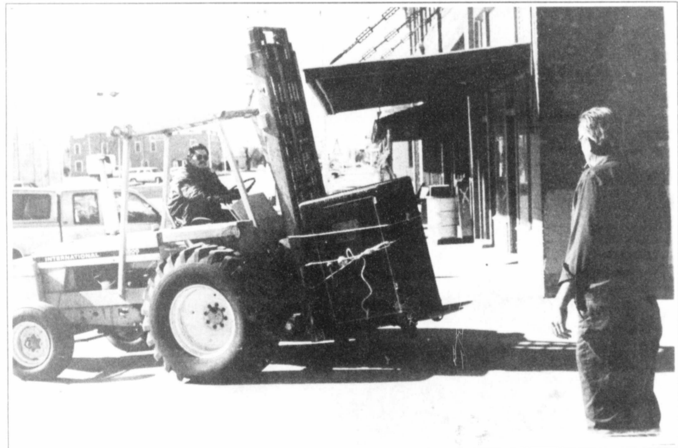
ANTIQUE SAFE CHANGES HOME--The old Surginer and Sons' Mosler safe was moved into The Hesperian-Beacon last week. The antique safe weighs approximately 3,000 pounds and was bought in by a fork lift from Brown Implement. The safe was originally housed in the Surginer & Sons building (now the Floyd County Historical Museum). It has been owned by several others before being bought by this newspaper from Joe and Juanita Stepp. The safe is in excellent condition except for the painting on the front door which was damaged in a fire in the Surginer building possibly in 1915. Staff Photo
