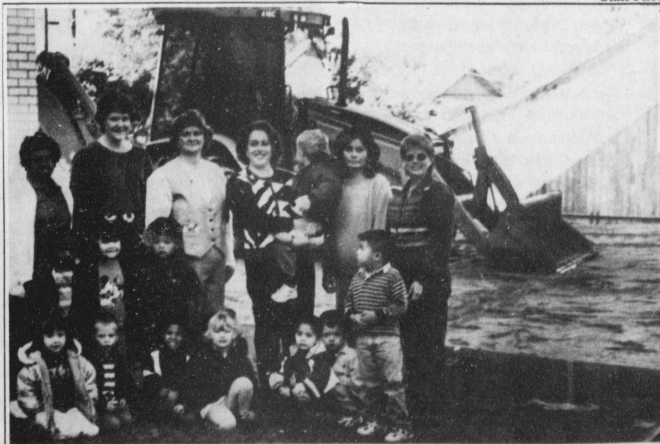
BUILDING A NEW DAY CARE --Some of the children from Floyd County Day Care took a trip to the site of their new Day Care Center which is being added on to the First Christian Church in Floydada. Work has already started preparing the ground for the foundation. Joining the kids at the site were Day Care Employee Carrie Davis, Board Members Dixie Smith, Gerry Summers, Jill Graham, Day Care Employee Aurora Johnston, and Board Member Denise Doucette. Staff Photo
