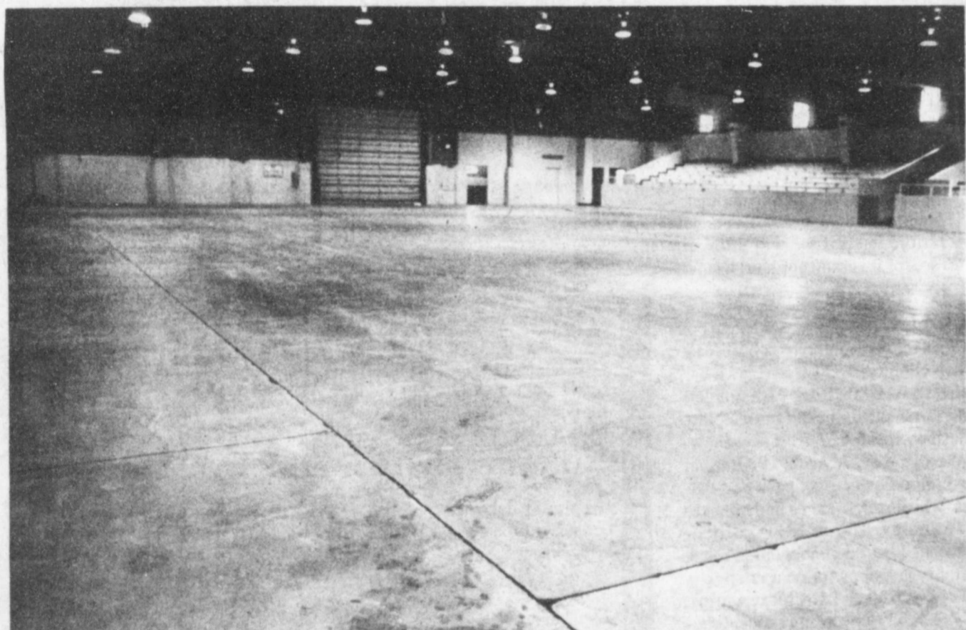
BAILEY COUNTY COLISEUM boasts of 18,000 square feet of covered concrete, permanent bleachers, storage, bathrooms and a 1,000 foot wash rack. This is a pattern that the Floyd County Friends hope to use in building the Multi-Purpose Center in Muncy.
