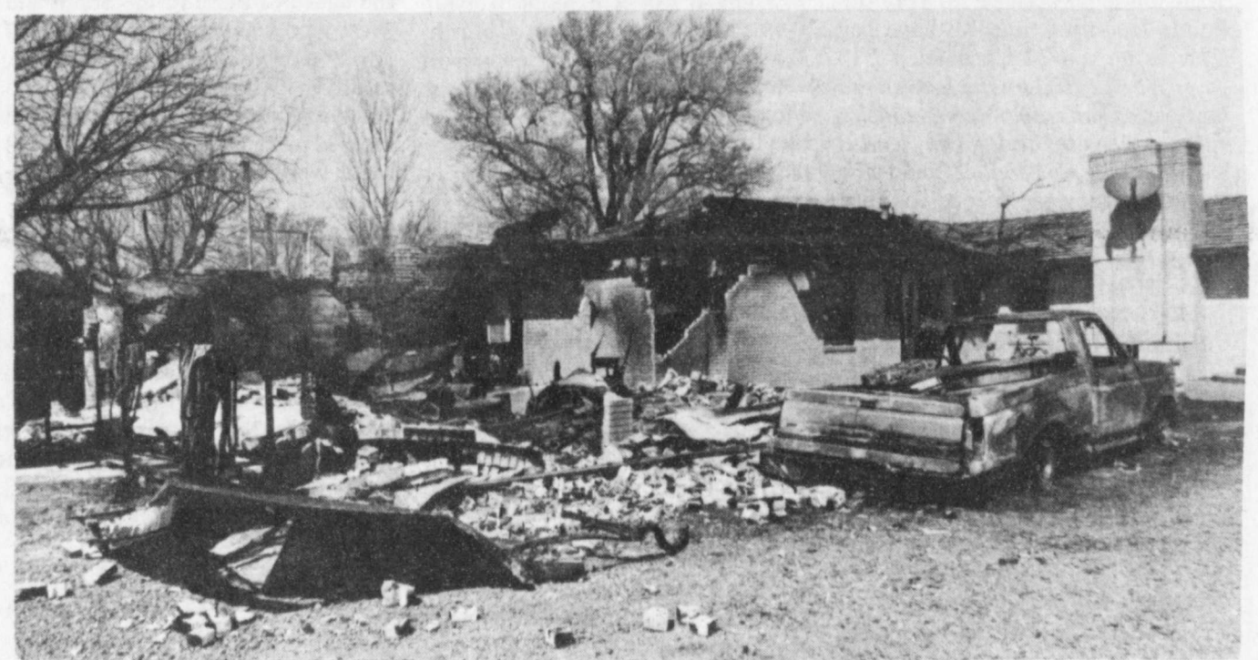
BELT'S GARAGE DESTROYED —A Monday night blaze destroyed the two story garage and pickup belonging to Johnnie Belt. The roof of the home was also damaged and the interior suffered smoke damage. Staff Photo
