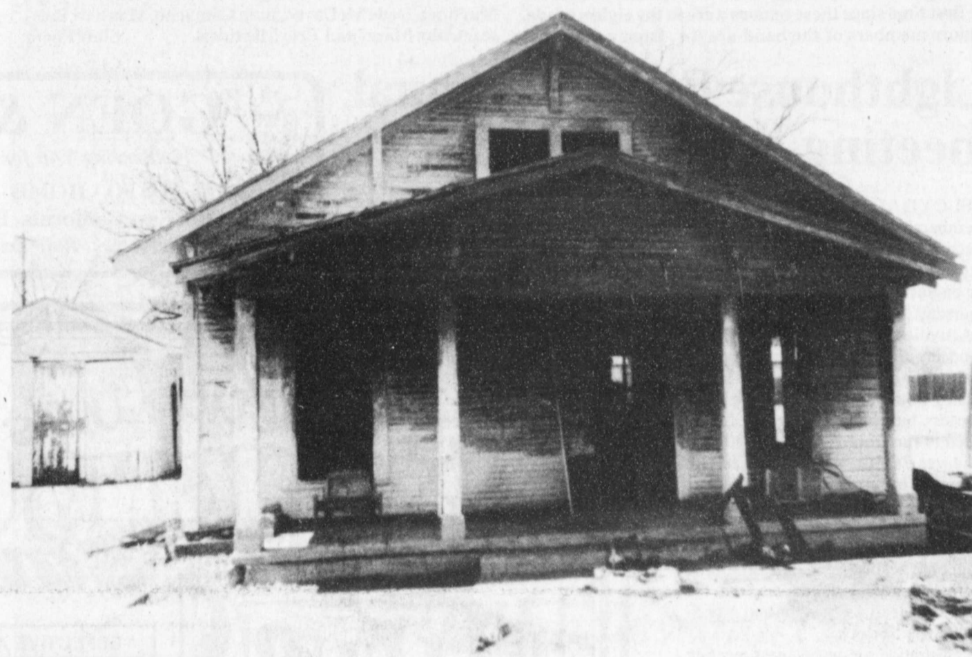
FIRE DESTROYS HISTORIC HOME-- The Jerry Workman home on SW 2nd Street in Lockney and all its contents were destroyed by fire in the early hours of Monday morning. Workman escaped by crawling through a bedroom window. The house was built in 1915 for John and Bettie Sams. Staff Photo
