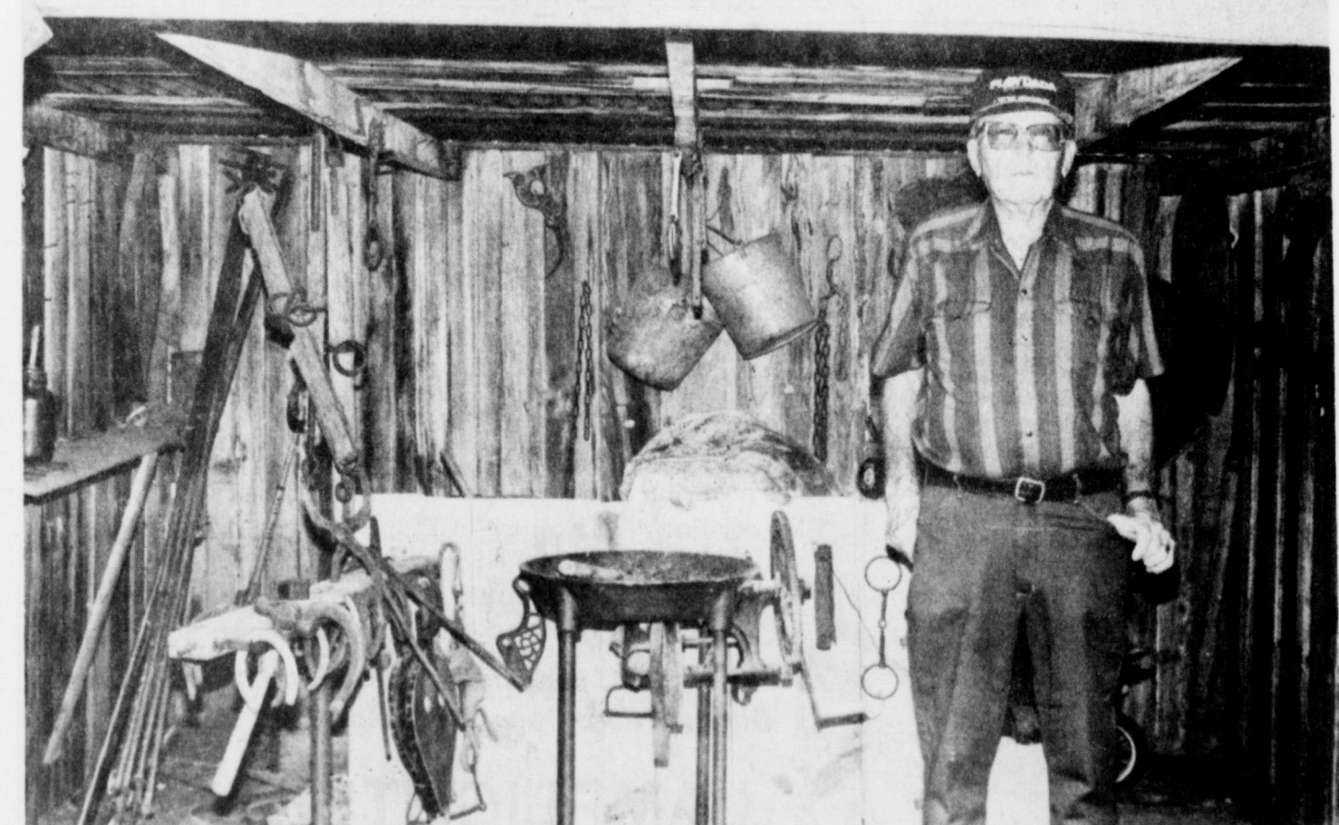
BLACKSMITH ROOM —Another room has been added to the Homestead to house all the tools necessary for blacksmith work. A.C. has old horseshoes, an anvil, billows and a forge containing coal for heat.
