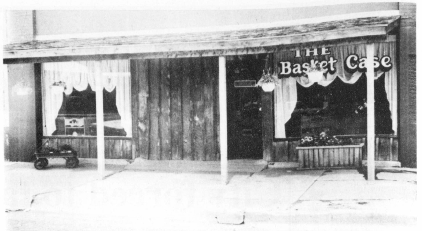
GIFT SHOP EXPANDS--The Basket Case, located at 103 South Main, Lockney, has added on extra rooms and a portico. The addition has given them more space and the portico enhances the front of their building. The owners,
